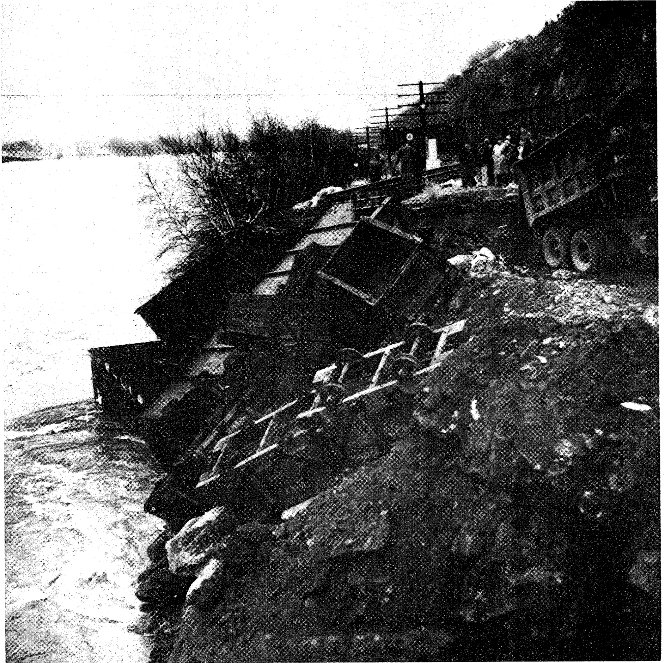
FIGURE 2. - Materials Being Dumped Into River Break-In Area.
