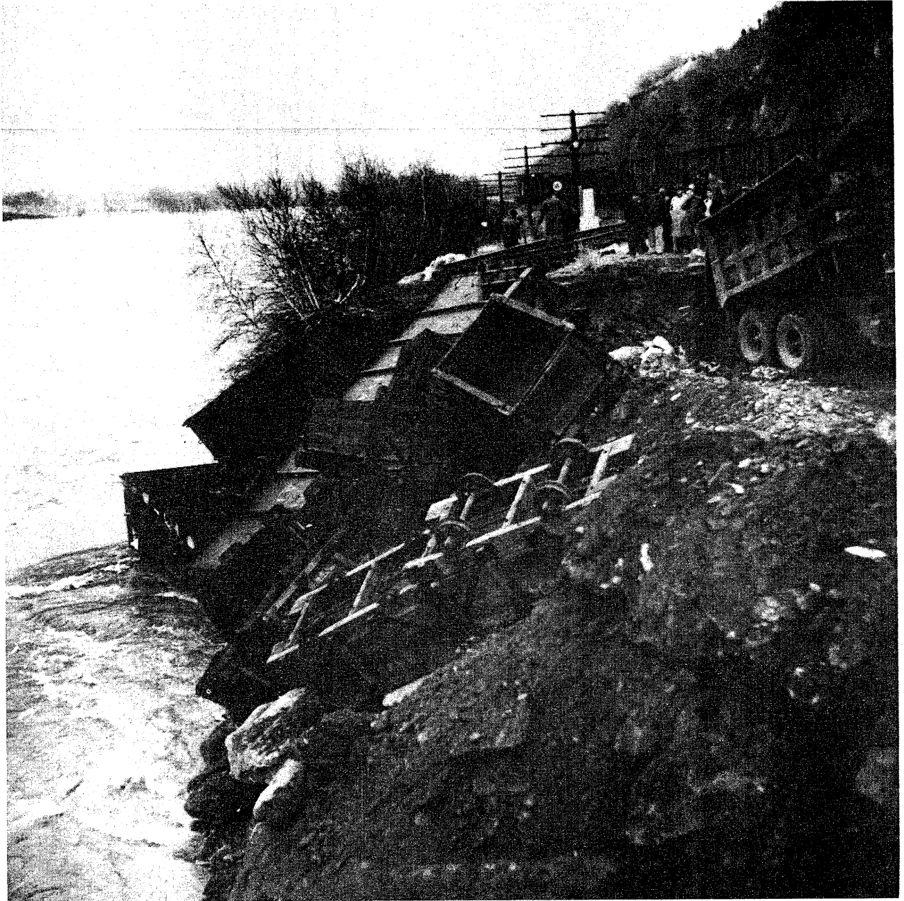
FIGURE 2. - Materials Being Dumped Into River Break-In Area.
