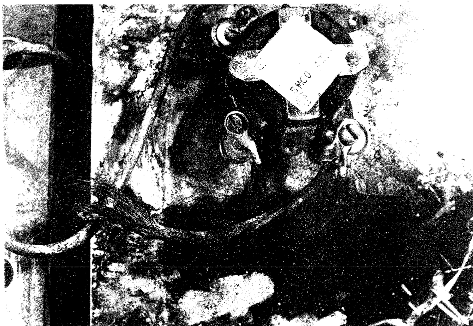
FIGURE 3. - Light switch and No. 14 wire inside McJunkin Corp. lighting system box.
