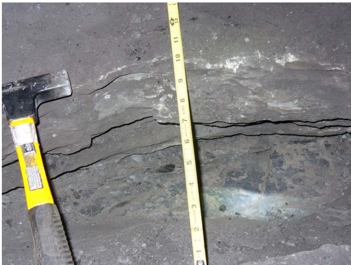
Figure Q-6. View of exposed floor heave crack looking straight down, with hammer and tape measure for scale. The crack is rootless and dies out approximately 12 inches into the floor at a layer of shale.
