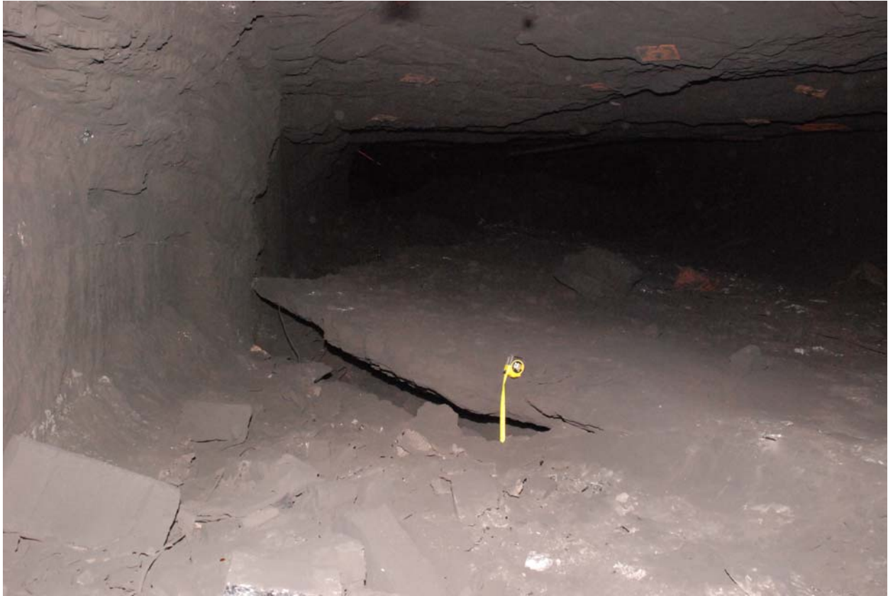
Figure 13. Cantilevered slab of floor sandstone forms broken brow with rootless, open aperture fracture. This style of floor heave is typical throughout Tailgate 1 North, the Panel 1 crossover and adjacent rooms, TG 22, and HG 22.
