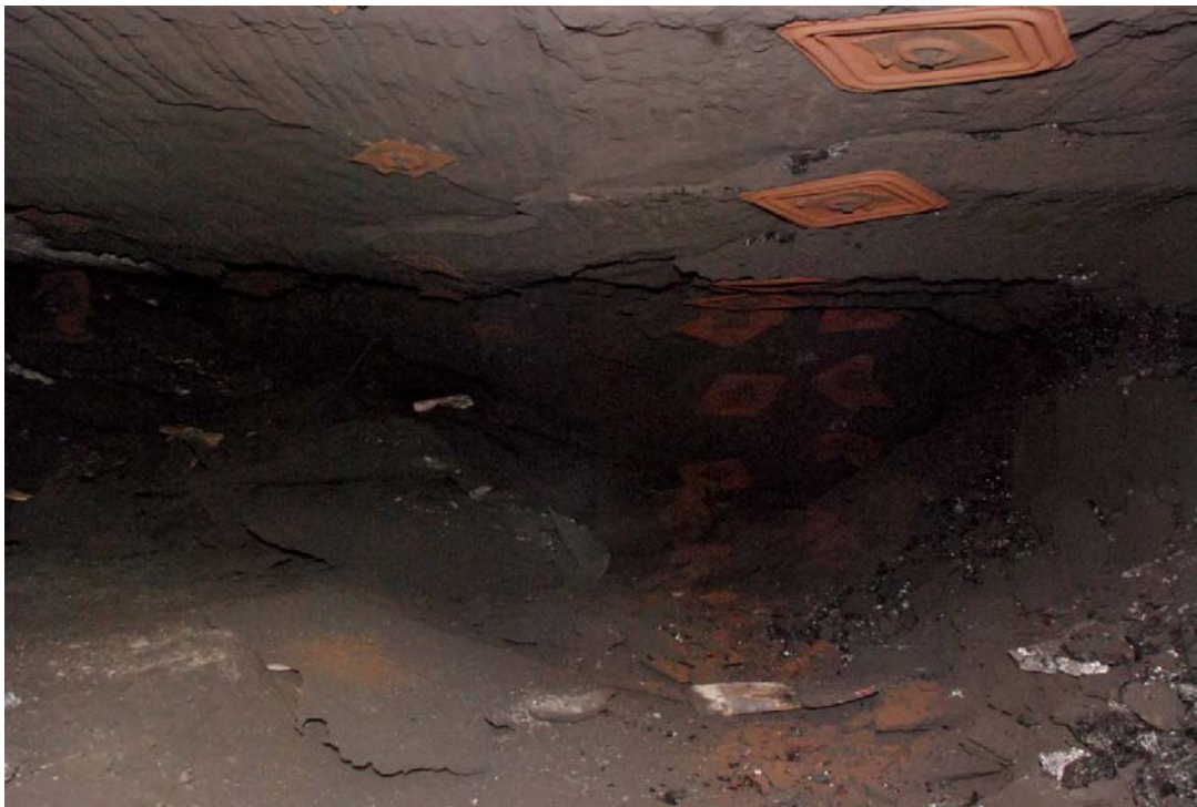
Figure 23. Caved roof in tailgate entry, as viewed in crosscut 49, which represents the next crosscut inby the face. Coatings of soot on the fallen rubble, juxtaposed against small pieces of freshly fallen, white sandstone, indicate that the intersection had caved prior to the explosion.
