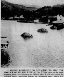
A BRIDGE DESTROYED BY LOYALISTS TO STOP THE ADVANCE OF SPANISH REBELS. The D'Onofre open on the main highway from San Sebastian to Bilbao, after it was destroyed by loyalist forces retreating before an insurgent army which had scored a succession of victories in the Bay of Biscay sector.
