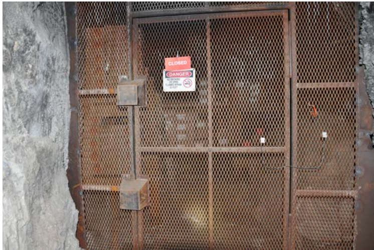
Figure 12 – Entrance to Powder Storage Facility
