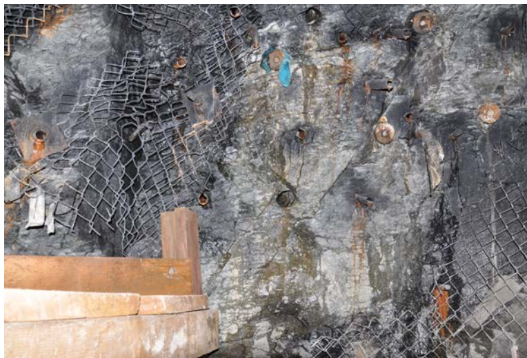
Figure 13 – Inside of Powder Storage Facility
