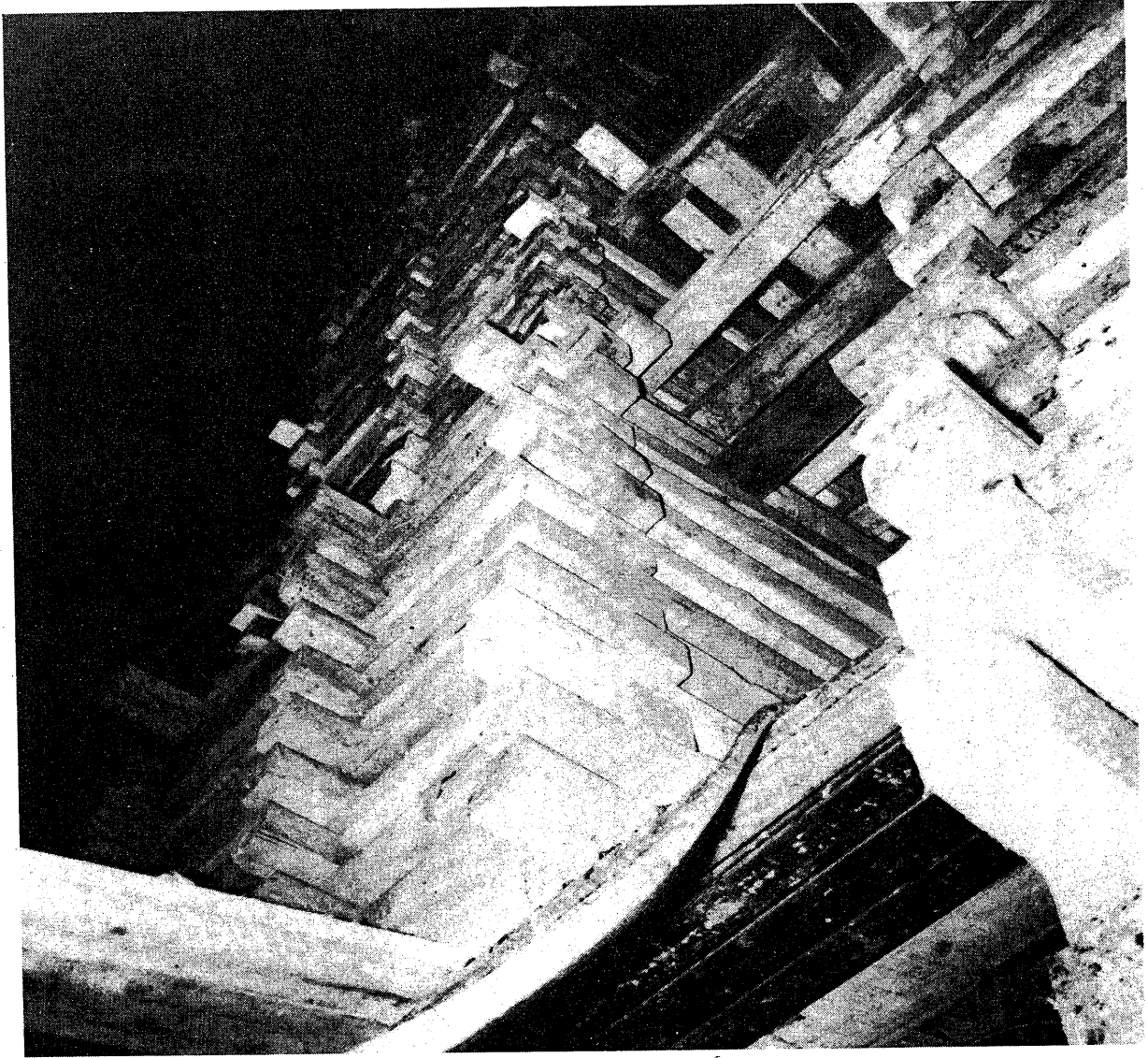
Figure 10. - Timbering in fire area.
