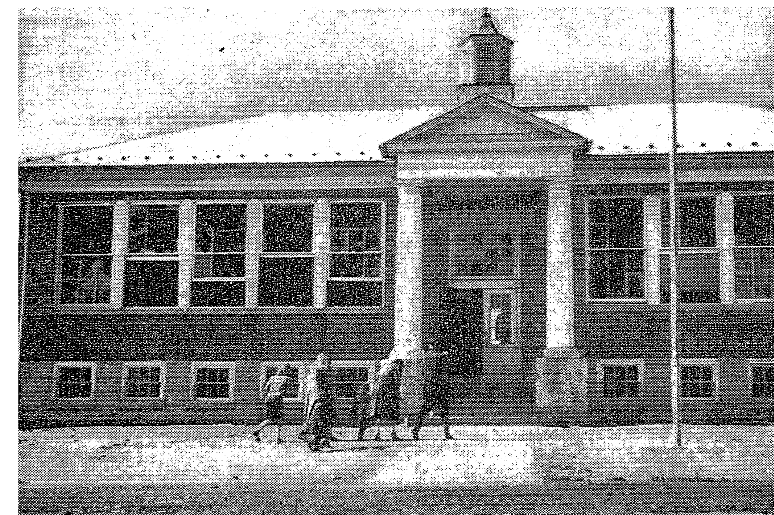
The Lehigh Consolidated School at Mud Run, about a mile southwest of the quarry, where sixty-one children were blown out of their seats. Note windows shattered by the force of the blast.
