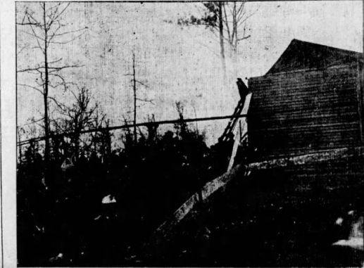
THE DAMAGED FAN HOUSE ABOVE THE MOUTH OF THE MINES AT VIRGINIA AND PART OF THE WING CROWD.
