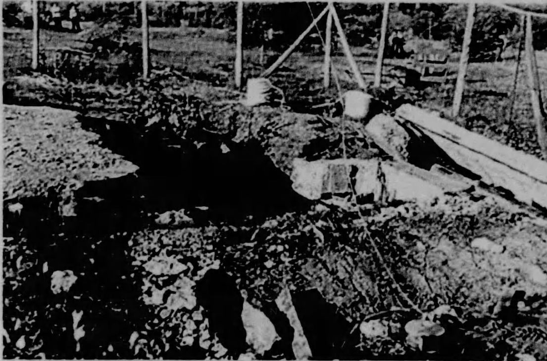
A 1966 photo shows the open mine pit where Ruth Ann Miller, 7, fell while playing with her brother, Gary, 10. The mile-deep vertical shaft is cluttered with debris, assorted timbers and pipes. The cap is shown at left. About half of the slab was broken to enable search operations. Submitted by Michigan Technological University Archives
