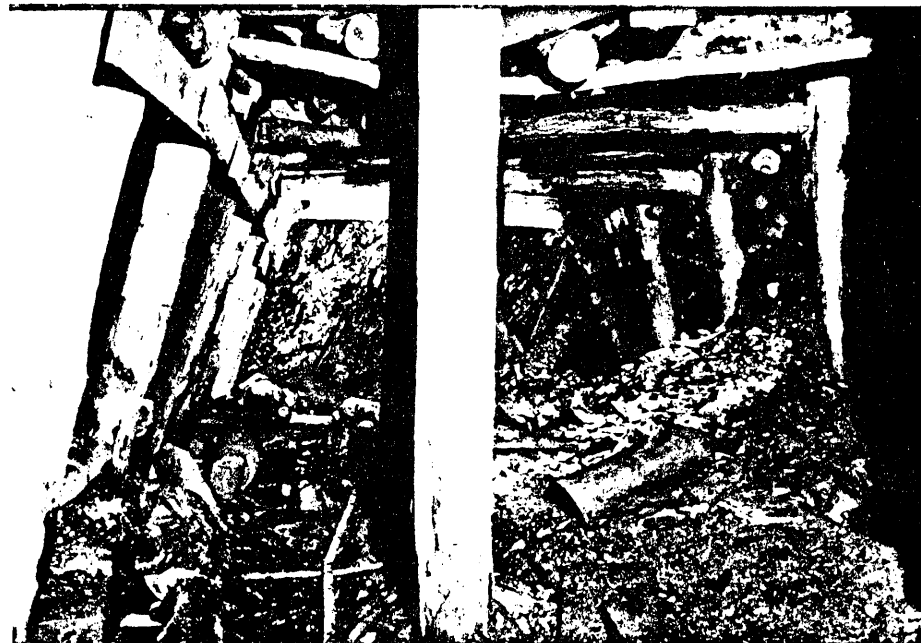
FIGURE 12 - Photo showing the timber and forepoles placed in the face area of the gangway during the rescue and recovery operations. View looking west.
