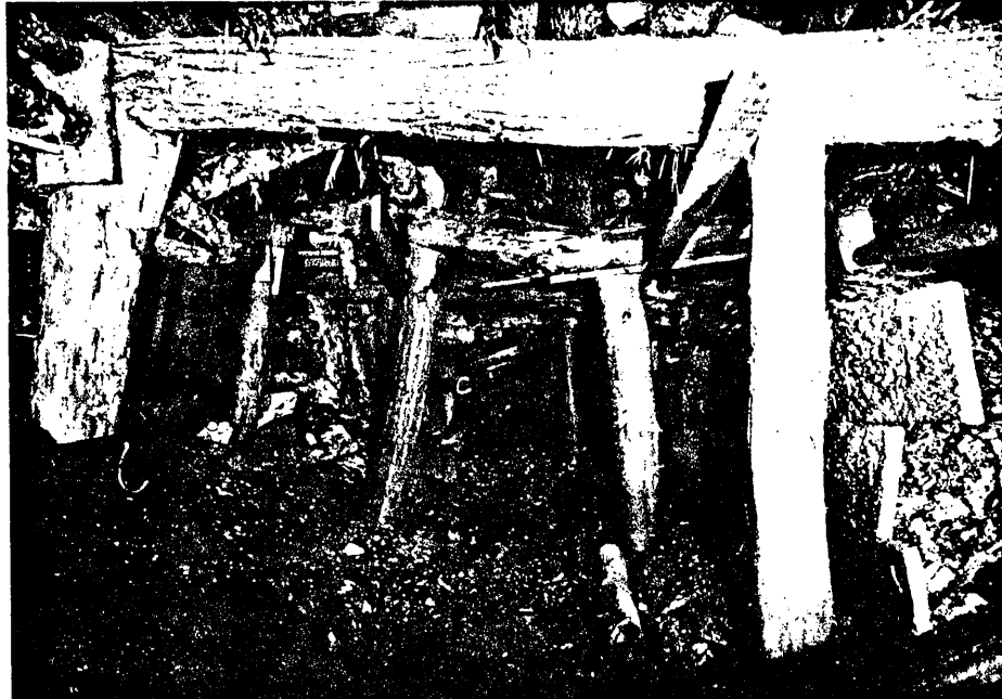
FIGURE 3 - Photo showing the condition before cleanup between Nos. 12 and 13 chutes in the gangway. View looking west.
