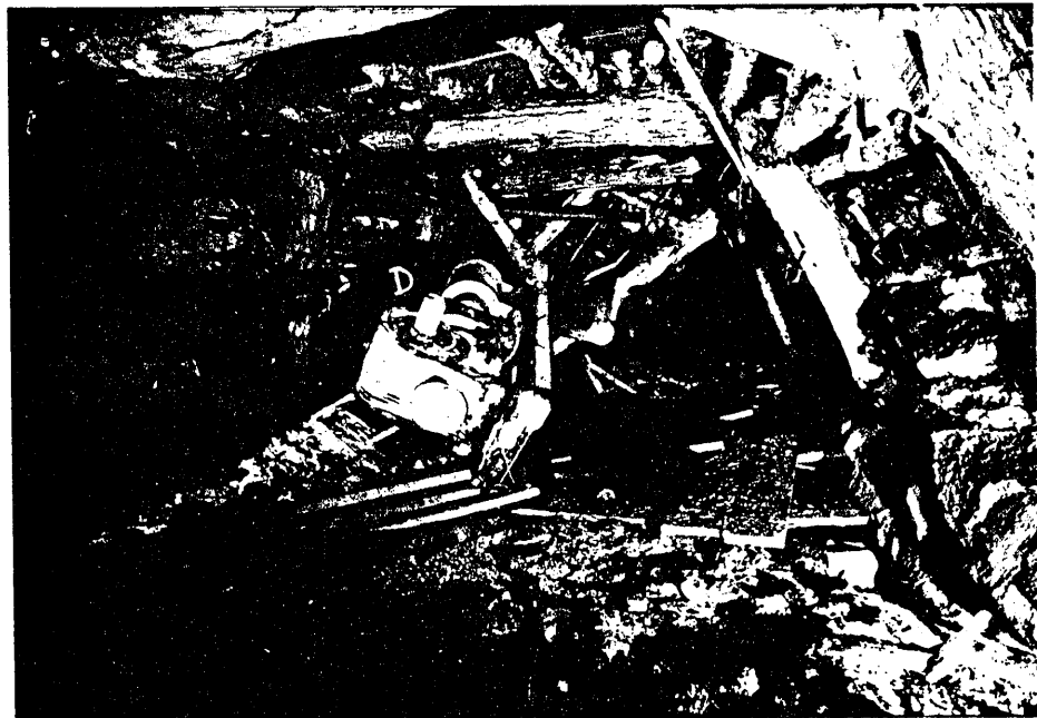
FIGURE 4 - Photo showing the overturned condition of the No. 2 conveyor drive unit located between Nos. 11 and 12 chutes in the gangway. View looking west.
