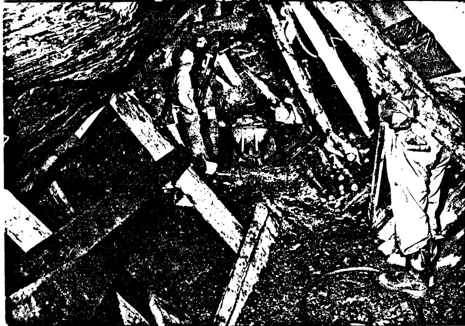
FIGURE 7 - Photo showing the face of the monkey airway inby No. 13 chute.
