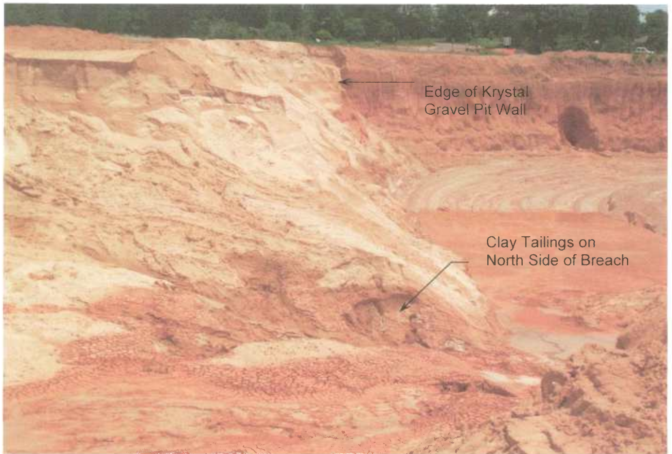
Photo 4 – View of the breach area and the eastern pit wall looking south. This view depicts clay tailings in the lower part of the pit wall on the southern side of the breach and the inside edge of the western wall of Krystal Gravel's Ball Pit in the background.
