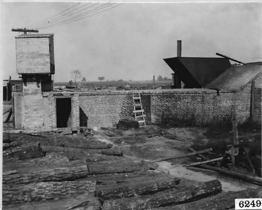
North Mine. Fire proof fan house and connections to the top of the air shaft.
