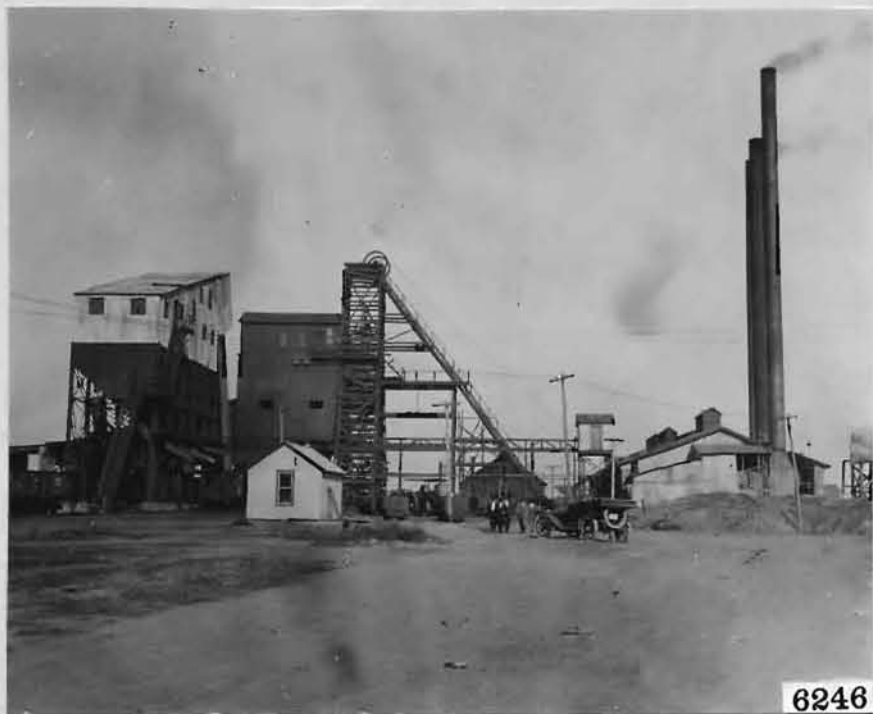
Royalton, Ill. Coal sizing plant. Power plant. Trolley and head frame.
