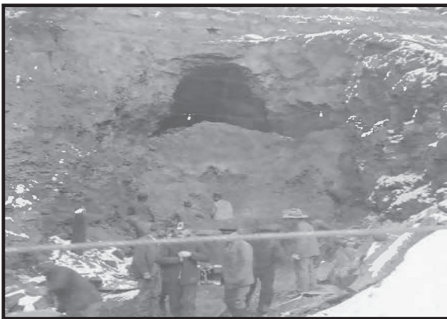
Men cleaning caved slope, Main North Mine
