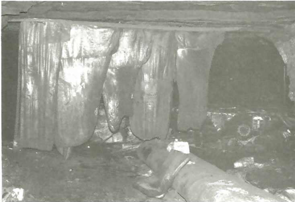
Fly curtain located in the No. 40 crosscut between the Nos. 3 and 4 entries.
