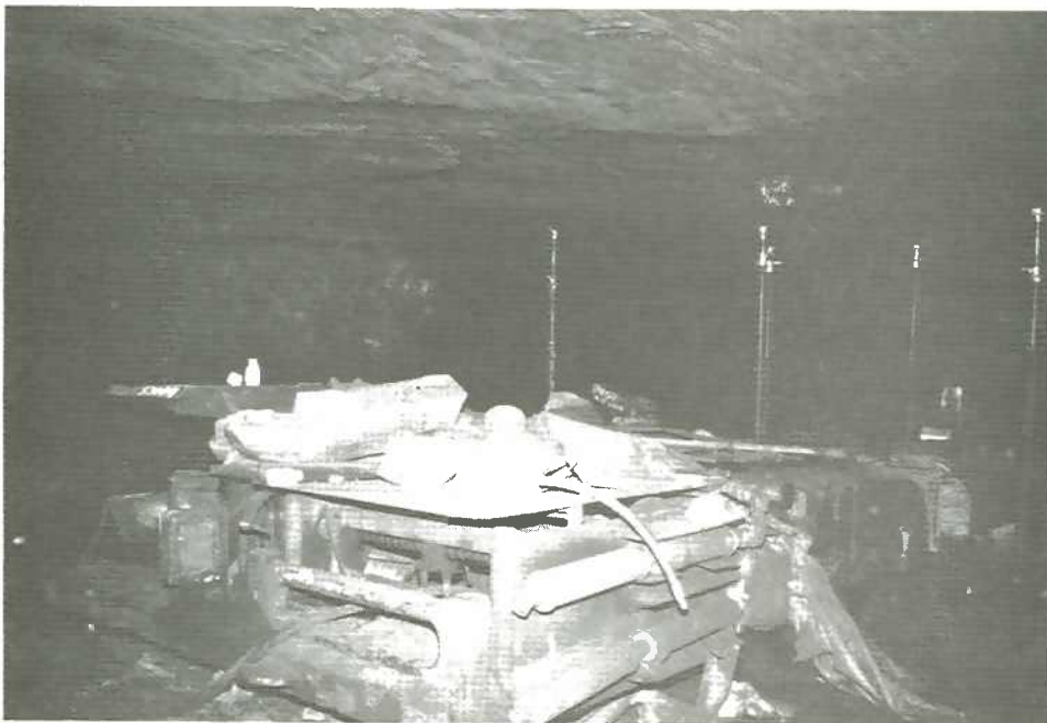
View of roof bolting machine located at the face of the No. 3 entry.
