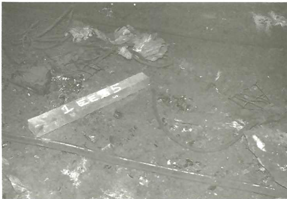
Portion of the power center lighting circuit and supply cable marked "Dinner Hole Lights" found 150 feet inby the power center.
